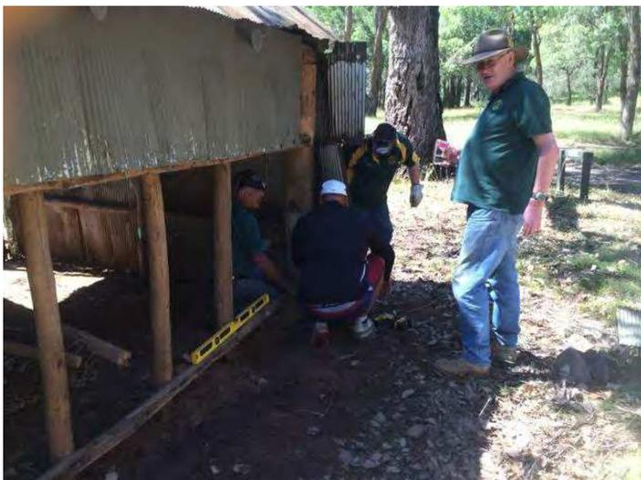
Photo: *The door being repaired and the tin being re-attached*
